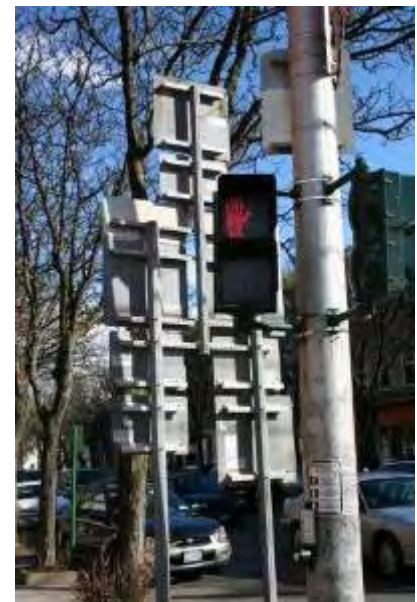
The City of Williamsburg, Virginia, to minimize sign clutter, clusters route shields (guide signs) on a single panel. On lower-volume roads the city uses smaller shields than on higher-traveled/higher-speed roads. Additionally, the backs of all signs in the city are painted to match the sign posts – minimizing the visual impact of signs when viewed from the opposite direction. Compare the Williamsburg route signs (left and center) to unpainted backs and individual shields (right) in New York. (Photos: Rick Taintor, Dan Marriott)
